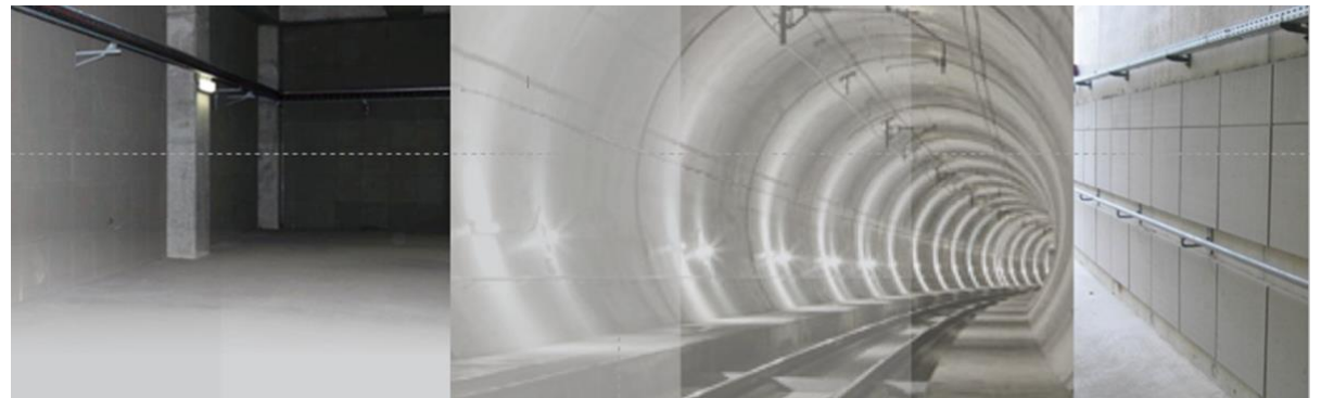
Tunnels & ventilation shafts
